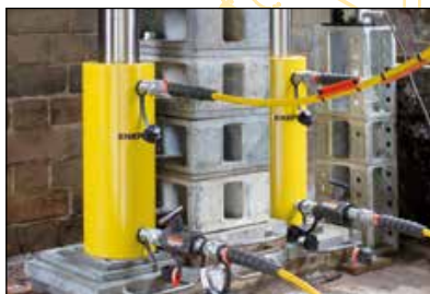
Bridge lifting and launching
