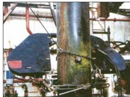
▼ Decommissioning job with band saw.
