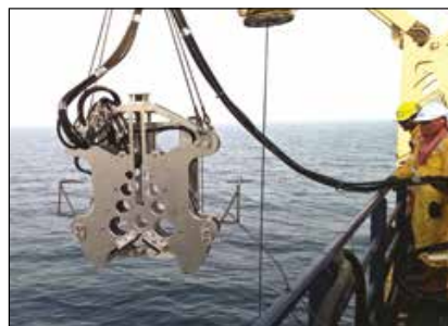
▲ MDWS Diamond Wire Saw lowered into sea.
