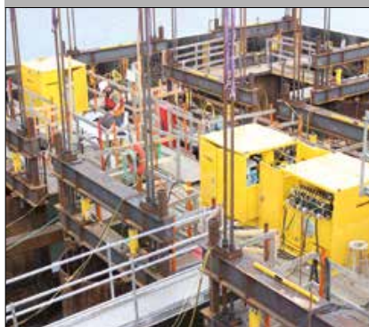
▲ Custom hydraulic pumps for a bridge deck launching system.
