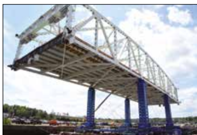
Incremental bridge lifting
