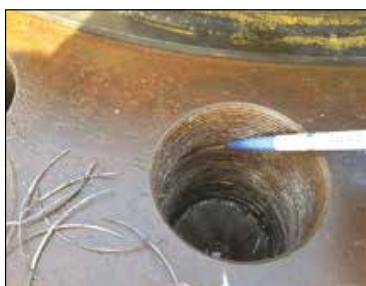
▲ A typical thread before refurbishment
