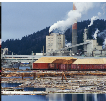
Slip Stream and By-Pass Sampling Filtration
