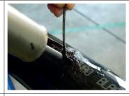
4.5 Spackle the melted material into the gaps by using a putty knife or similar. Make sure that enough melted material is used for the repair.
