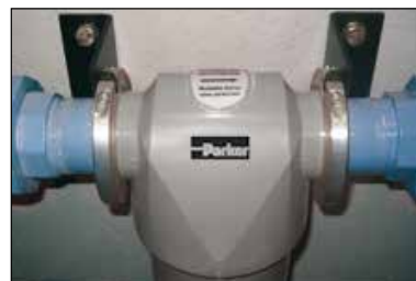
Wall Mounting Bracket Kit Mounting brackets provide additional support to filters installed in flexible piping systems or OEM equipment.
