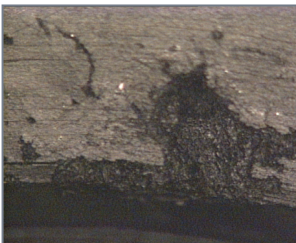
Pitting on filter end-cap
