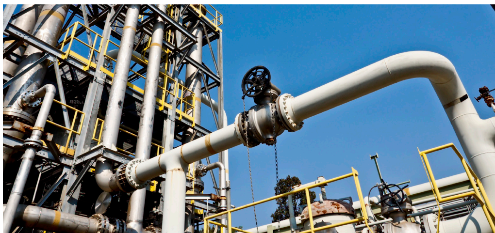
TAMAP Ultra low emission double block and bleed valve.
